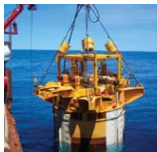
Installation of riser.
