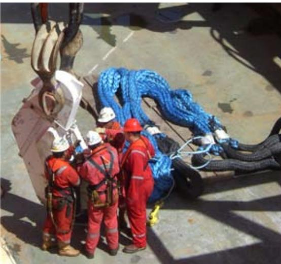
*Technip personnel "pre-rig" the hardware packages with the 88-mm AmSteel<sup>®</sup>Blue grommets.*
