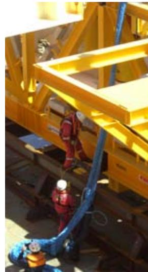
The use of a high-strength, "buoyant," sling was a must for this stage in the process. The hand off from the 400-metric-ton overboard crane to the A&R winch was simplified with the help of the AmSteel®Blue grommets. The foundation piles, pump stations, and manifolds were all "pre-rigged" before the over boarding process.
